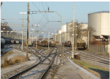
The nine-track Auhafen hump yard in 2013, before re-signalling. The project removed the connection between tracks 4 and 5 and renumbered all tracks. *Photo Bruno Huber*.
